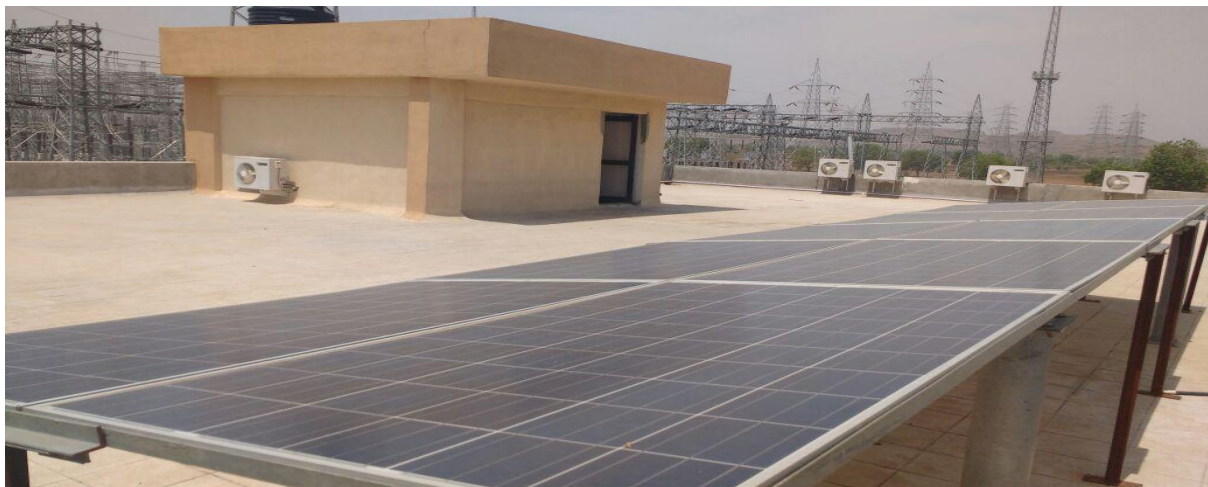
Roof top solar system at PGCIL substation , Aurangabad
