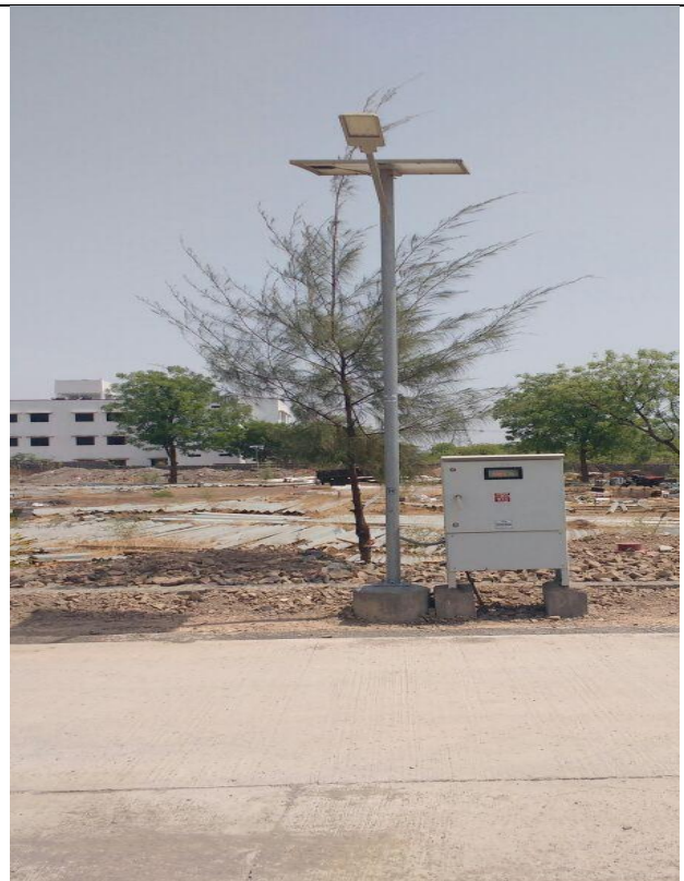
Site at PGCIL Substation, Aurangabad
