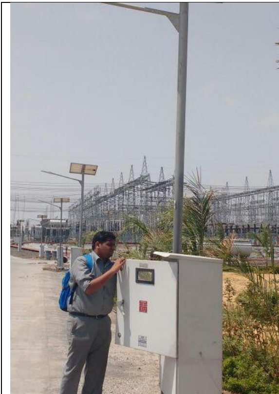
Site at PGCIL Substation, Aurangabad
